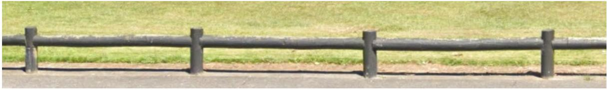
In ground H5 no.1's / 125 – 150mm diam/ Fix with 100 galv jolt head nails / or skew drill in 150 hex head galv screws
